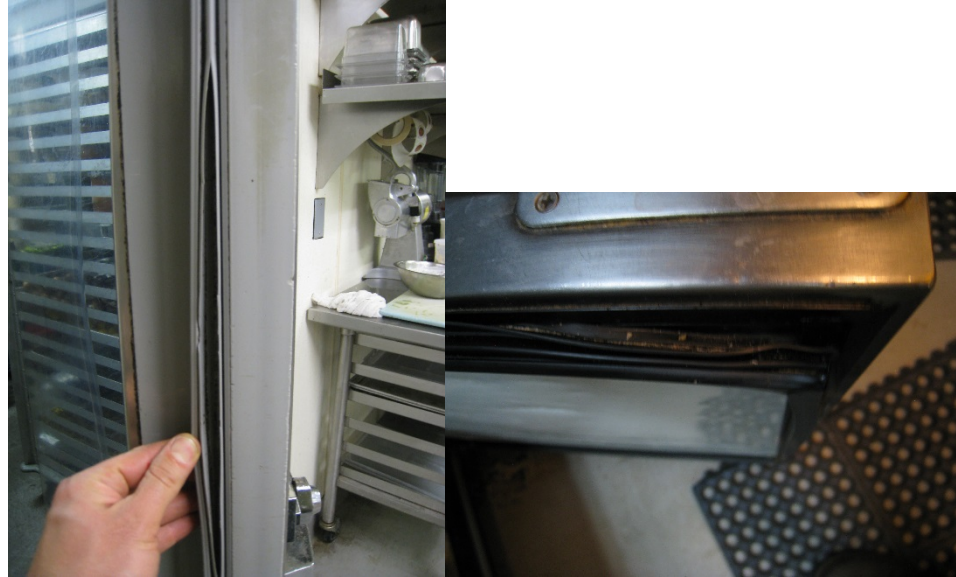
Figure 3-3. Installed Gaskets at Site 10
