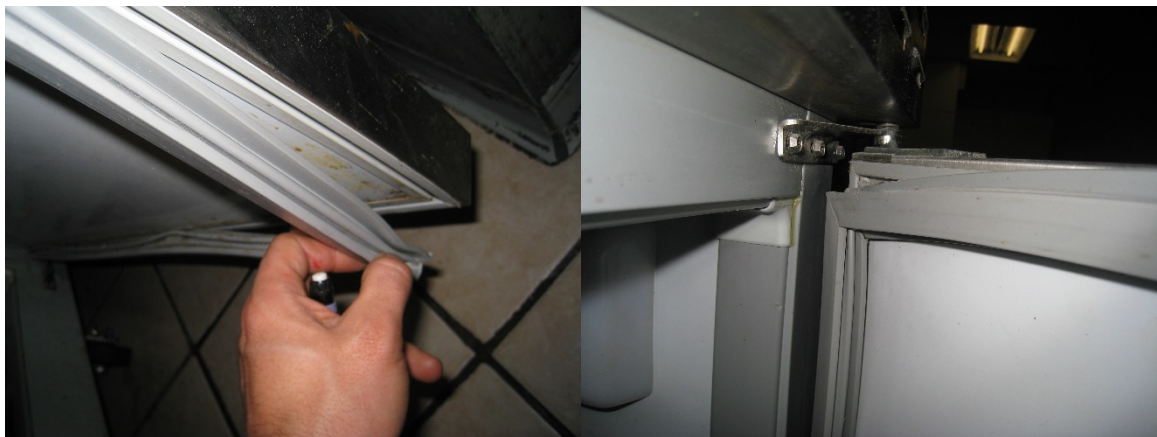
Figure 3-5. Installed Gaskets at Site 11
