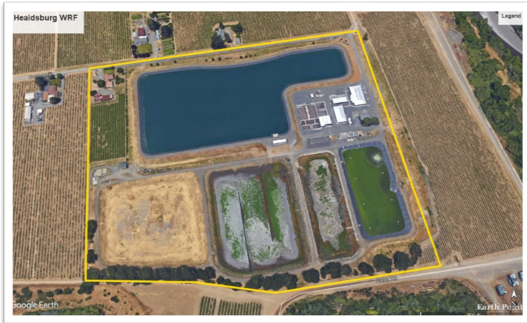
Figure 3.5-1 Proposed Project Site, Healdsburg Water Reclamation Facility
