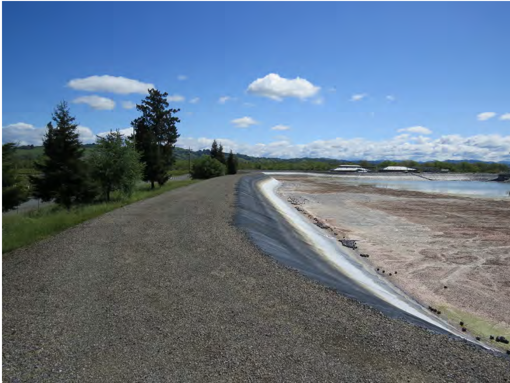
Photograph 3: From the northwest corner of the north pond looking east along the northern boundary of the pond.
