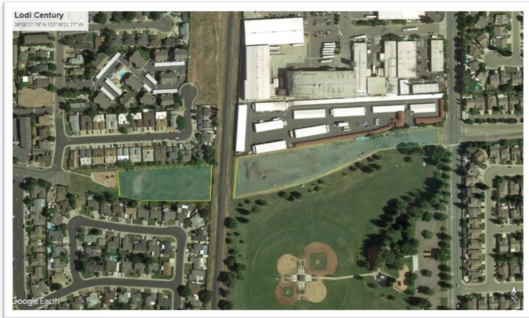
Figure 2 Century Park East/West Site
