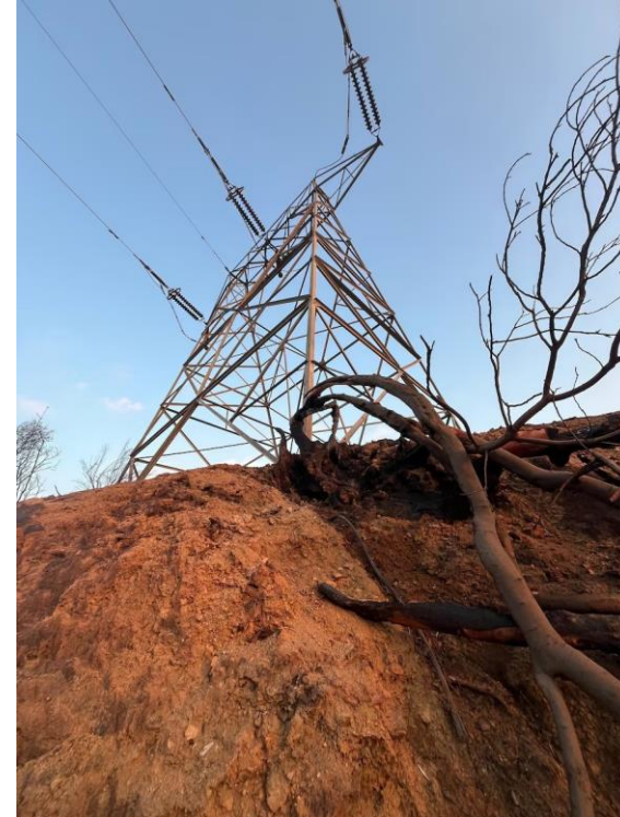
36kv tower and grounding wire, Eaton Canyon, January, 2025
