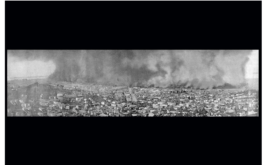
Fire following quake: the view from Twin Peaks, April 18, 1906.
